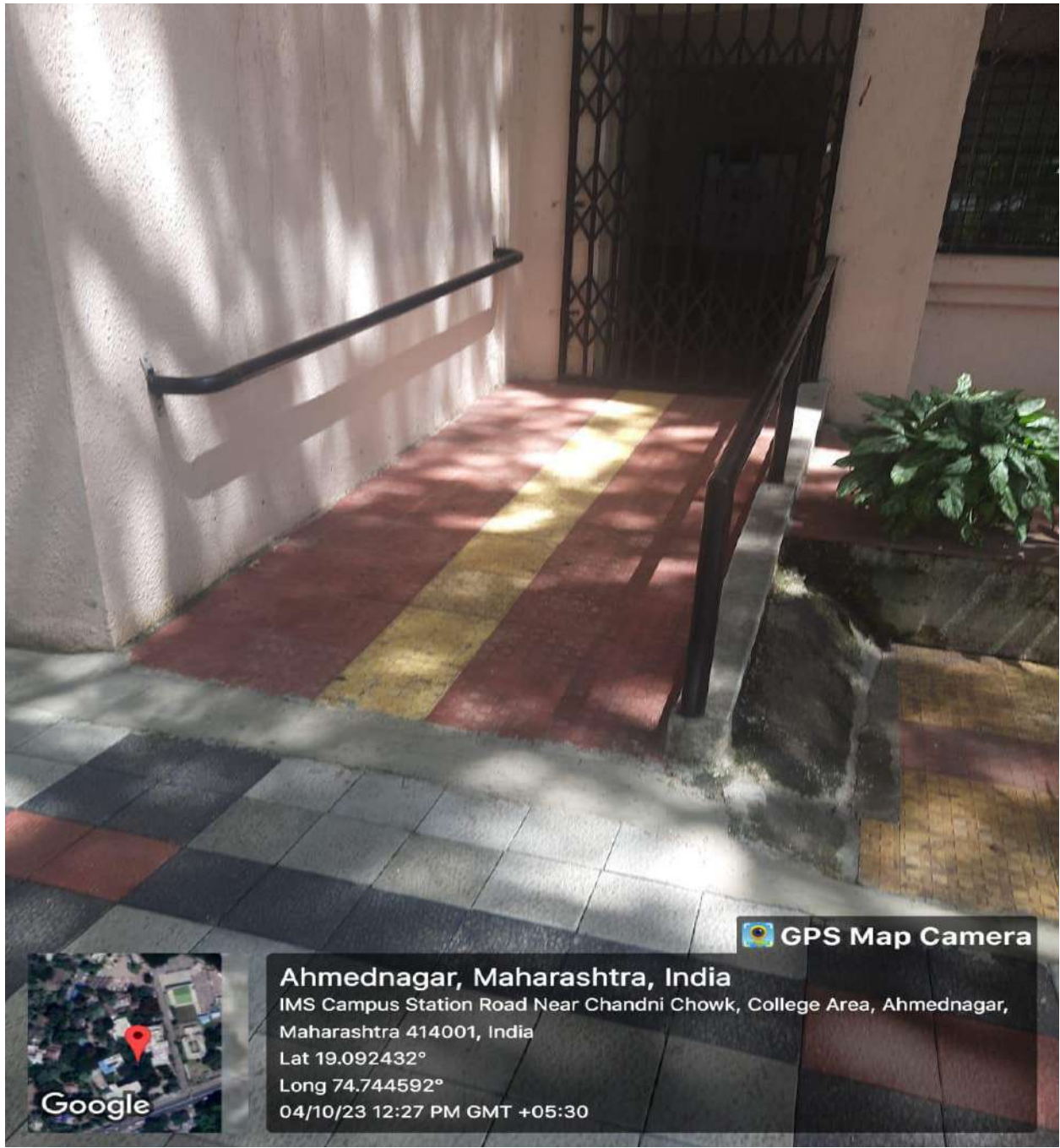
Disabled Friendly Ramp
